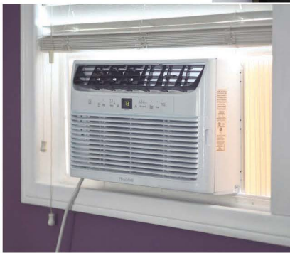
Make sure that your window A/C unit is installed flat or according to manufacturer's directions so that it drains properly.
